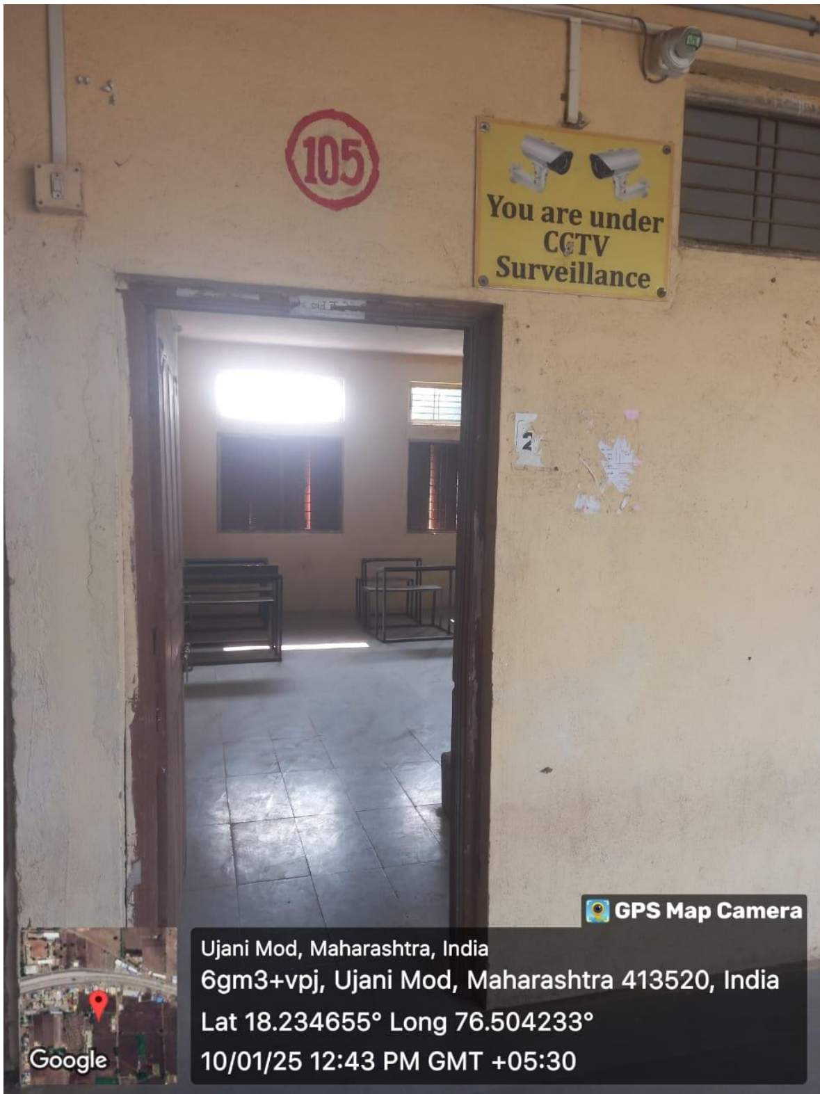
Class Room No. 105 (External view)
