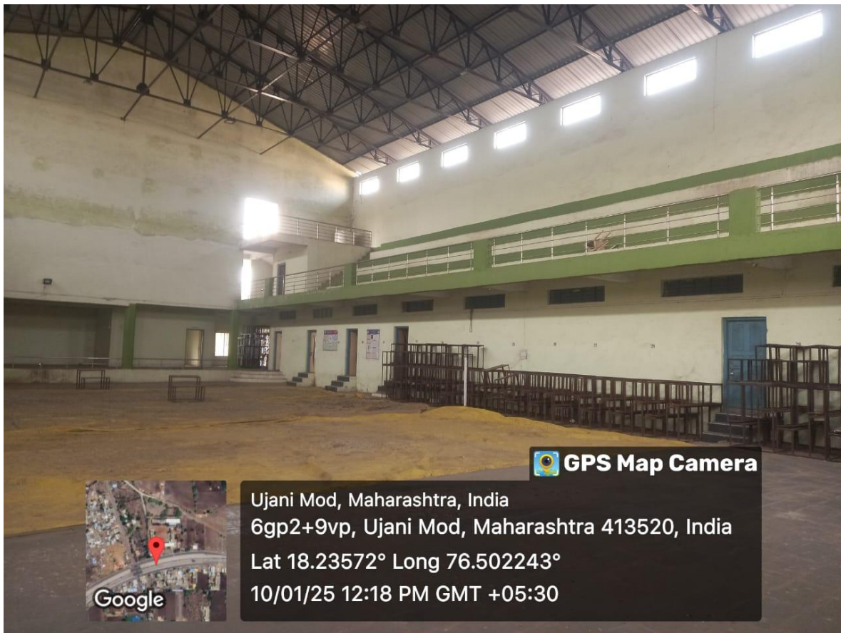
INTERNAL VIEW OF SPORTS INDOOR STADIUM
