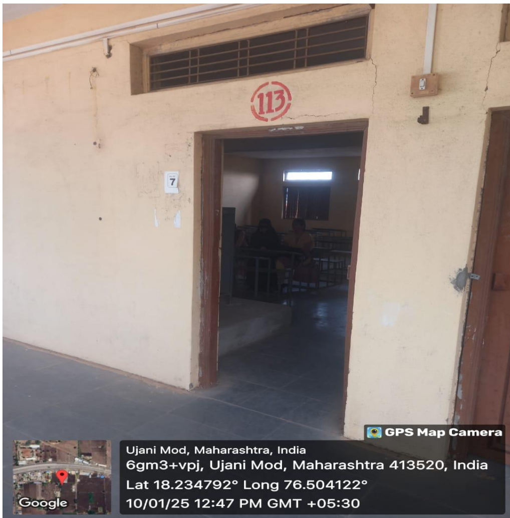
Class Room No. 113 (External view)
