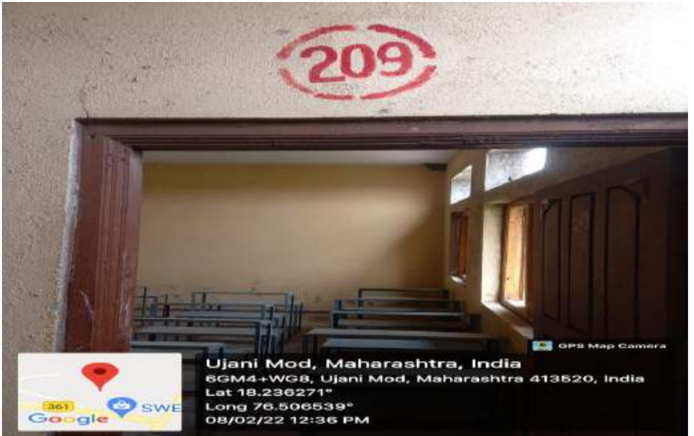
Class Room No. 209 (External view)
