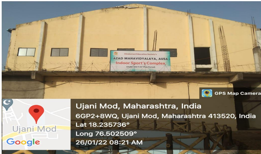
Front View of Azad indoor Sports Complex situated on North side of National Highway in campus II
