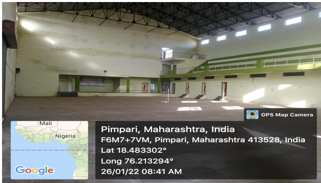
Interior View Azad Indoor Sports Complex Showing the Viewer Gallery
