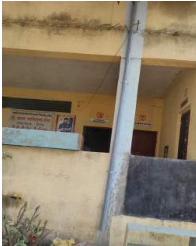
Completion of Rain water Harvesting System during lock down period (Covid)
