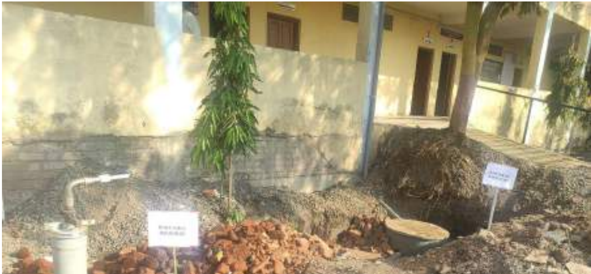
Installation of Rain water harvesting system
