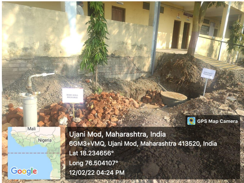
Bore Well & its recharge pit Photograph
