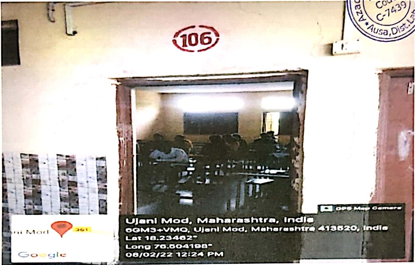
Class Room No. 106 (External view)
