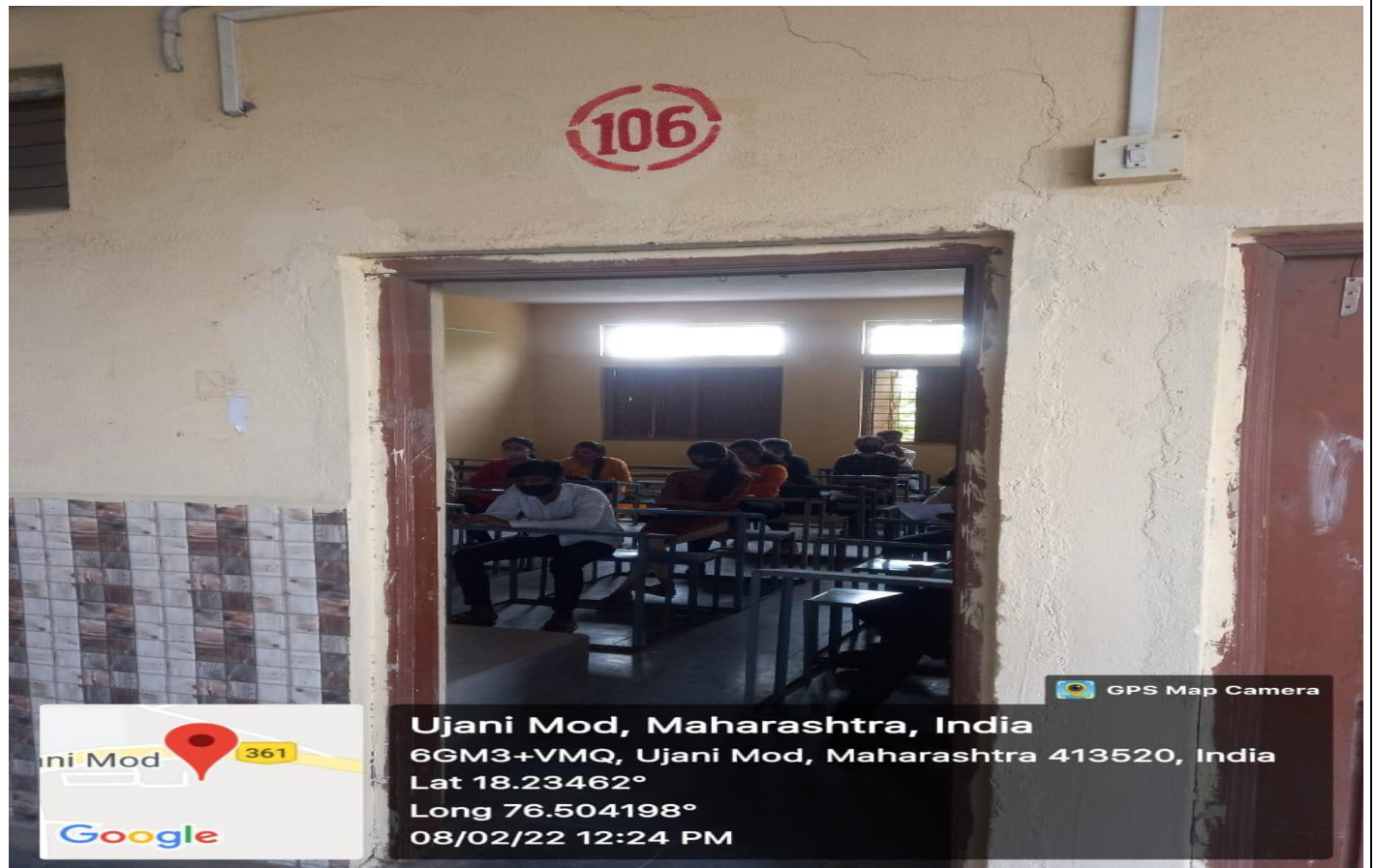
Class Room No. 106 (External view)
