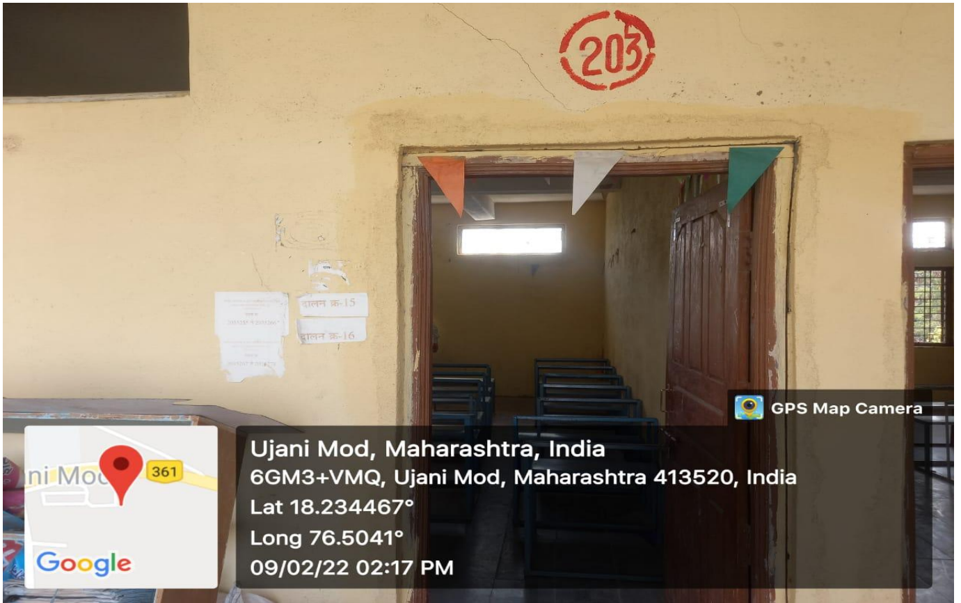
Class Room No. 203 (External view)
