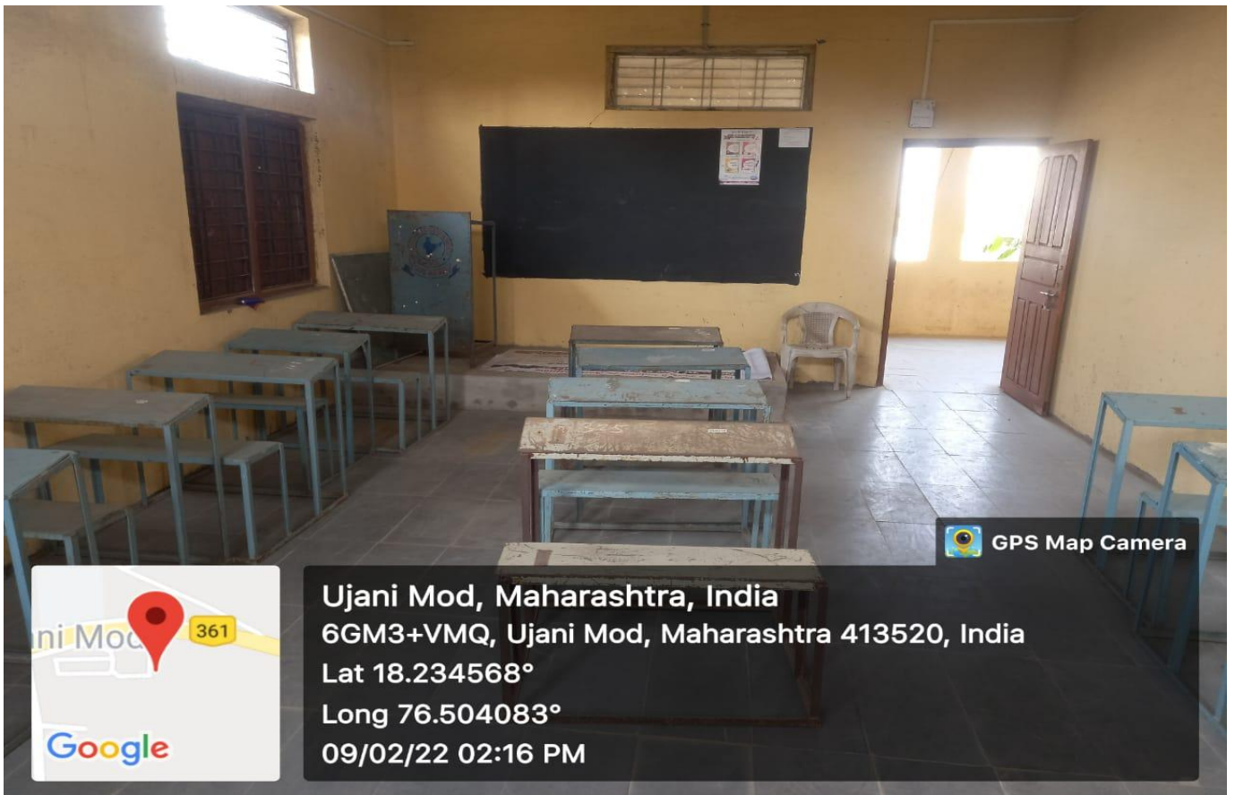
Class Room No. 202 (Internal view)
