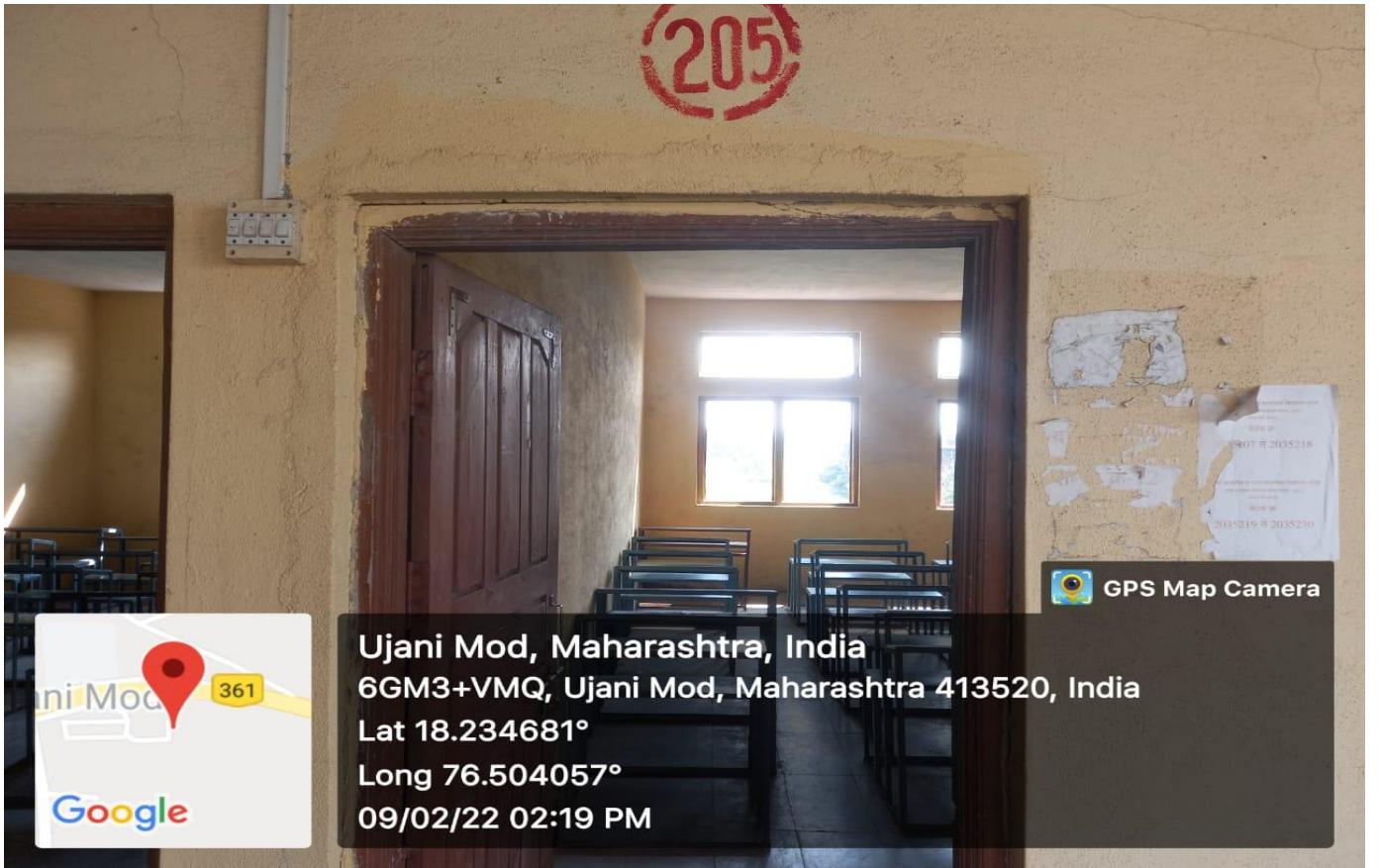
Class Room No. 205 (External view)
