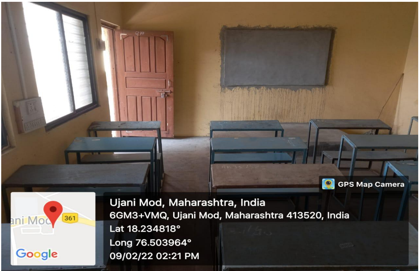
Class Room No. 210 (Internal view)
