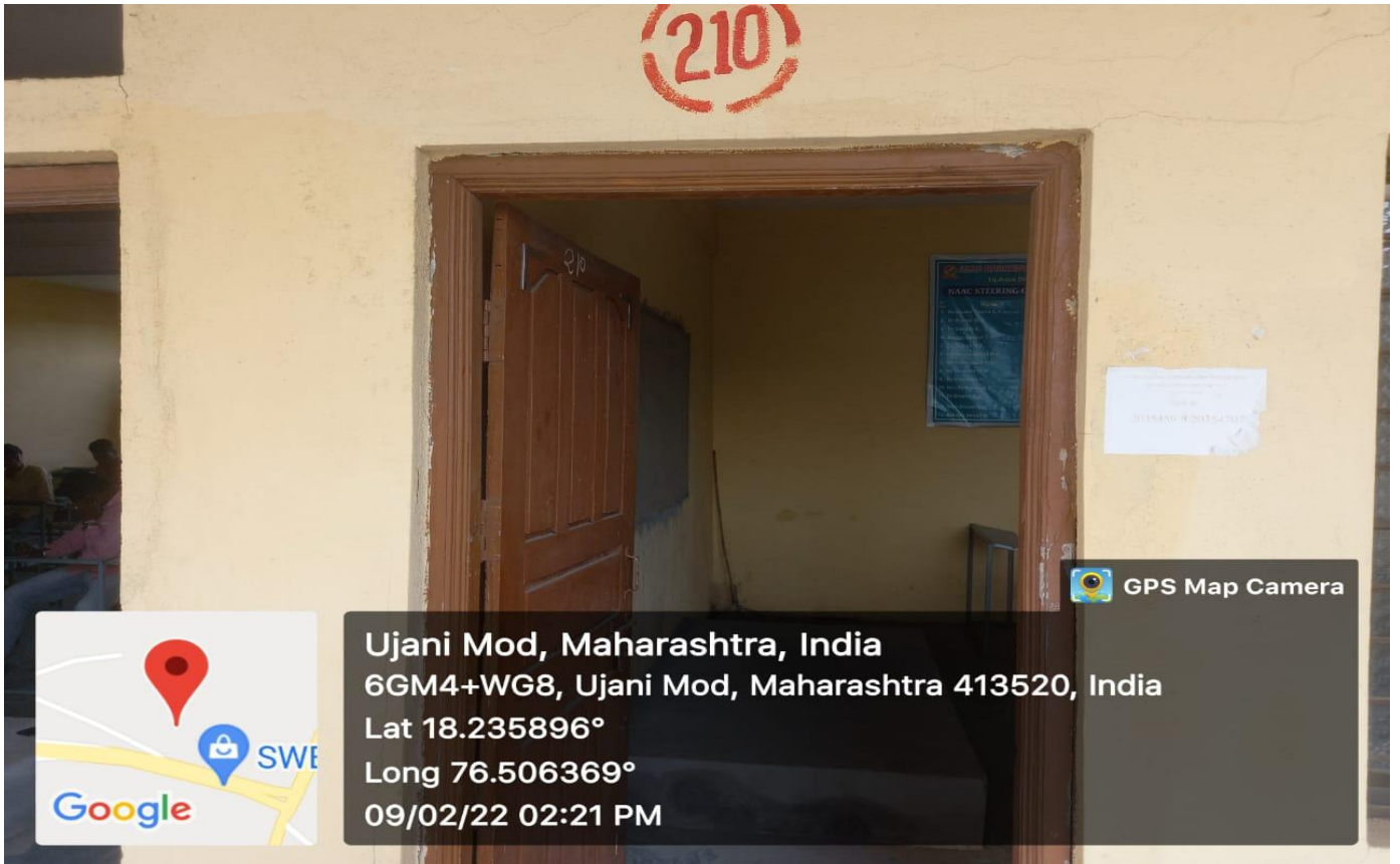
Class Room No. 210 (External view)
