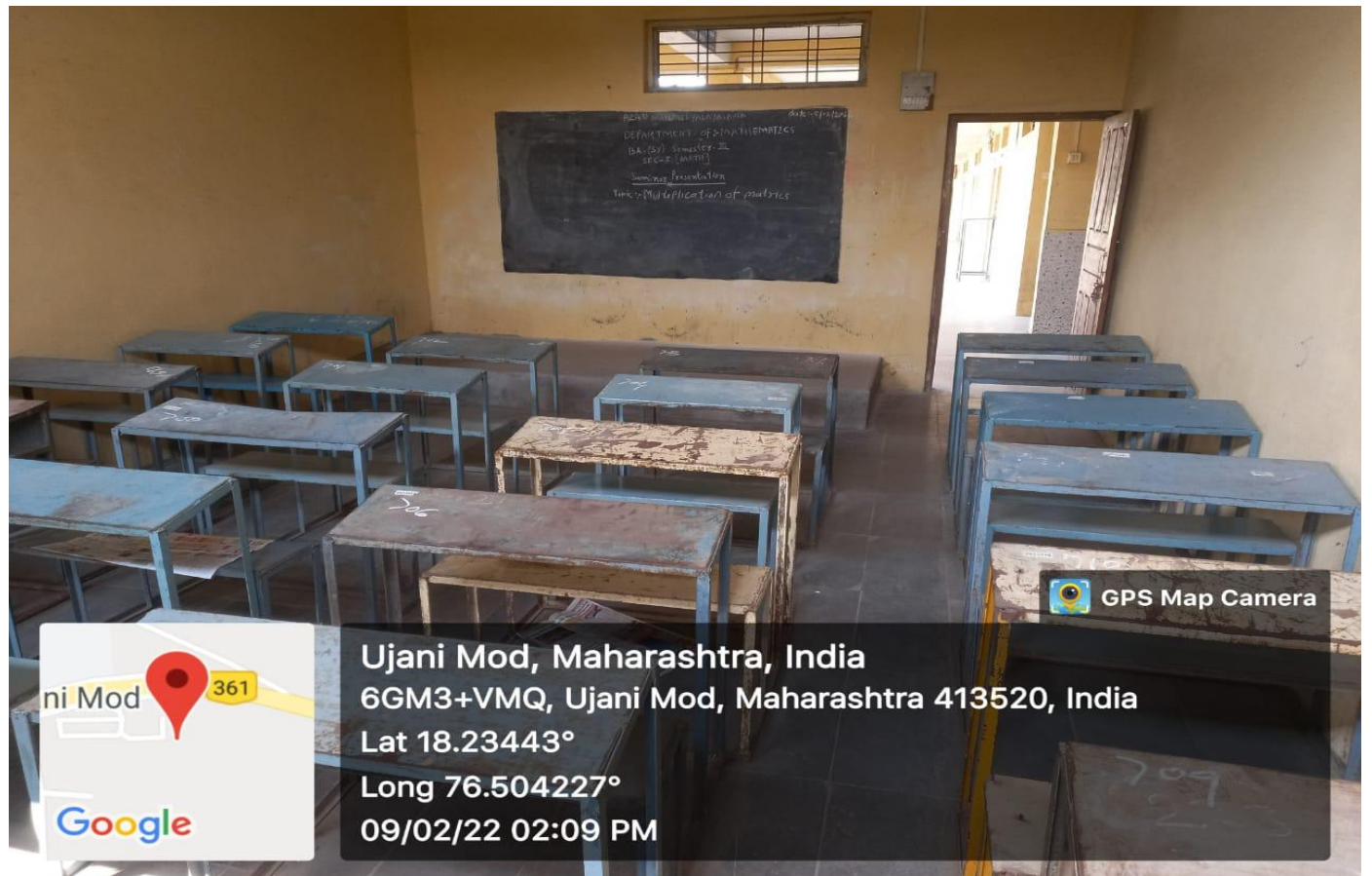
Class Room No. 105 (Internal view)
