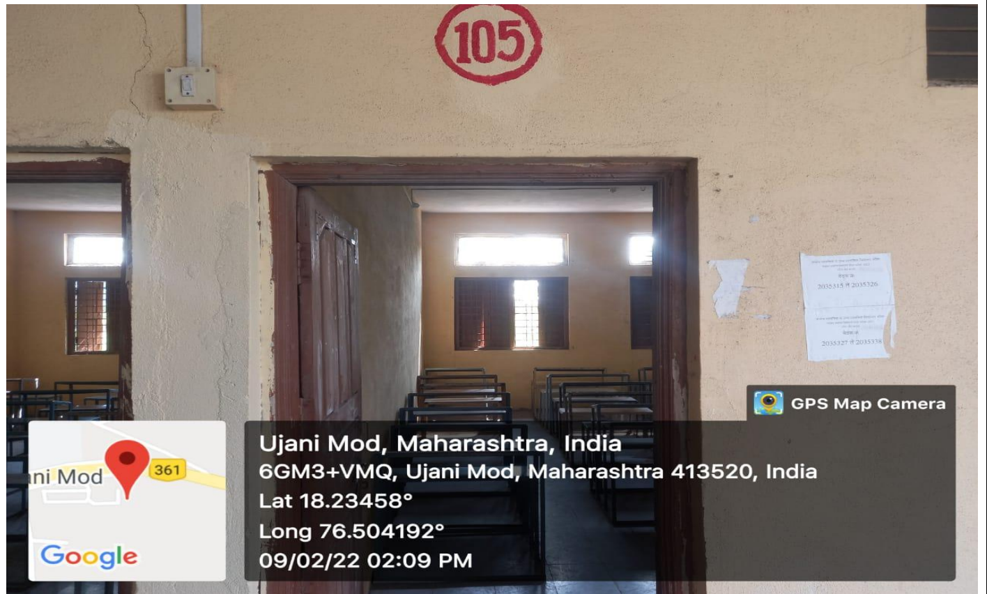
Class Room No. 105 (External view)
