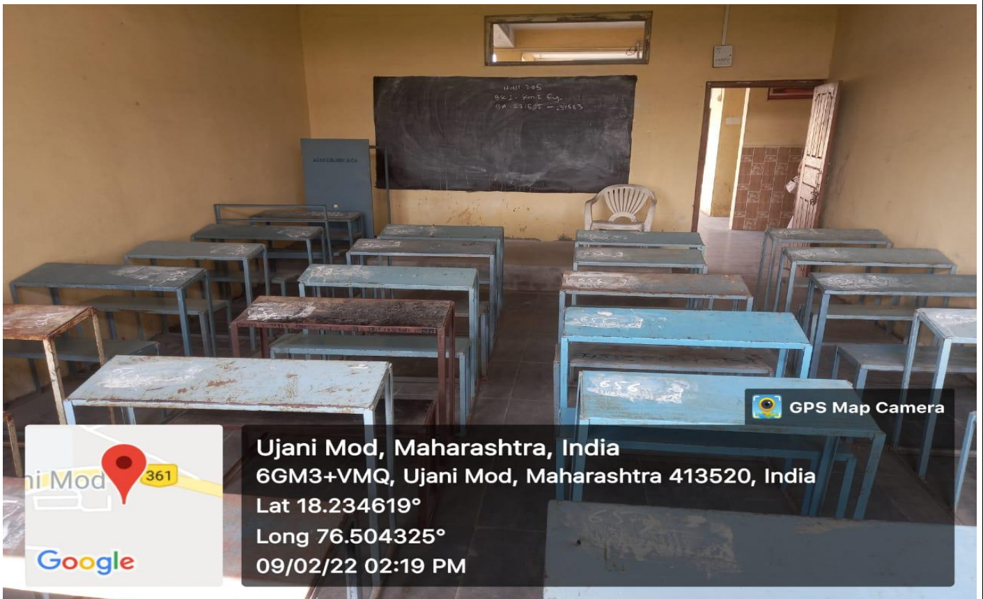
Class Room No. 205 (Internal view)
