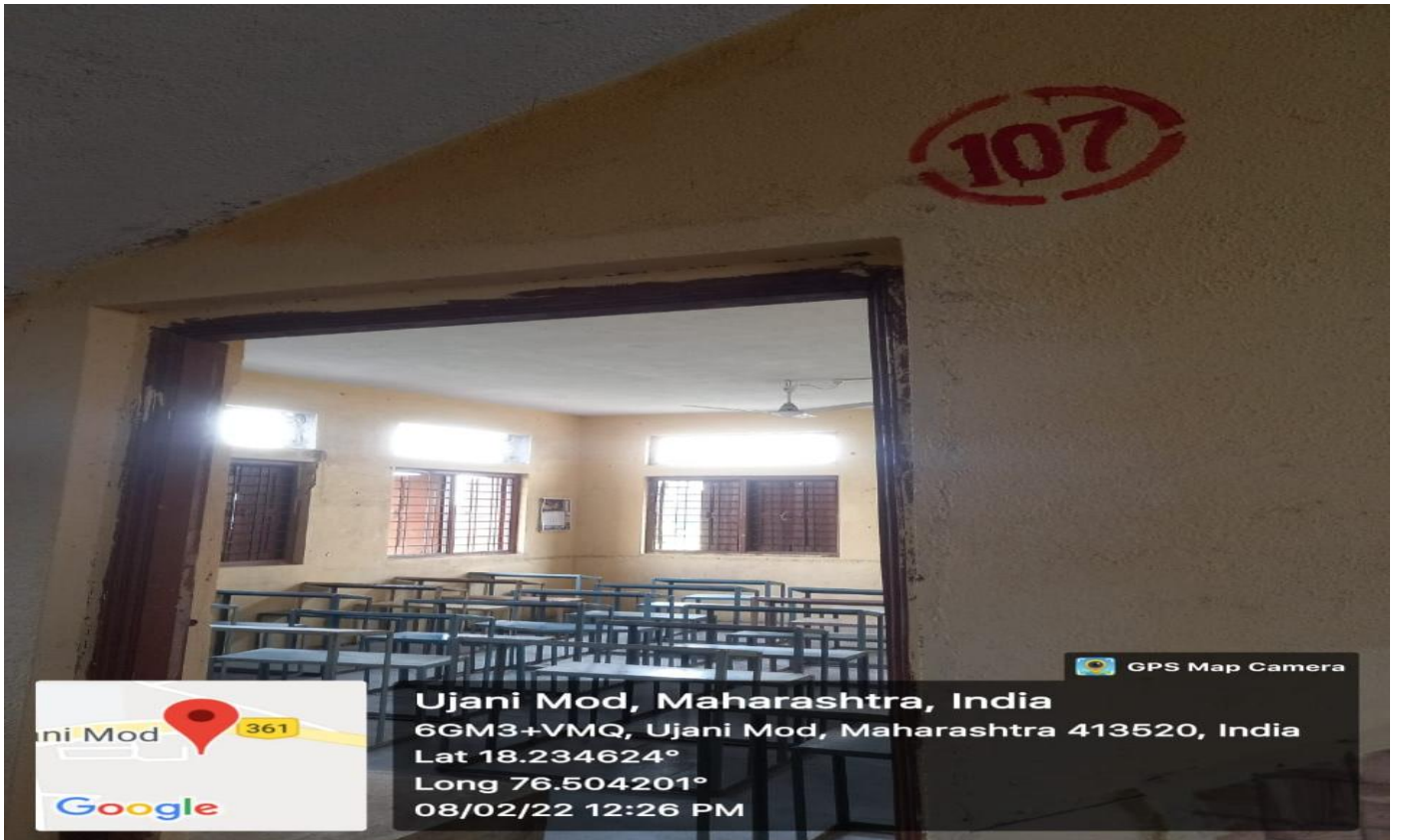
Class Room No. 107 (External view)
