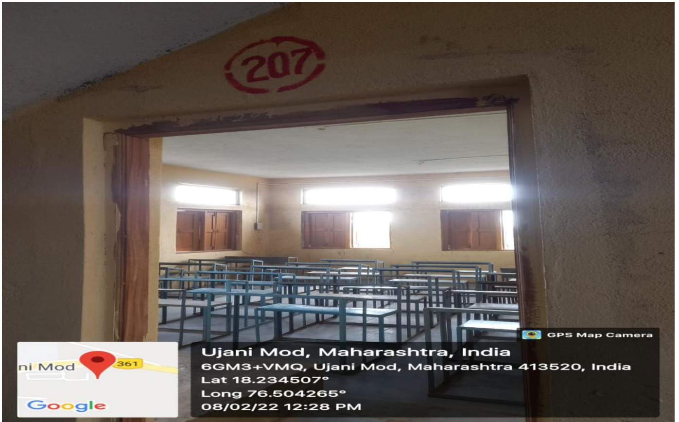
Class Room No. 207 (External view)
