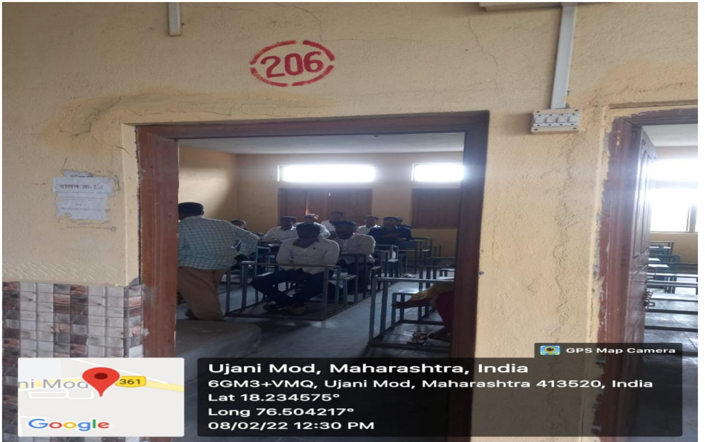
Class Room No. 206 (External view)
