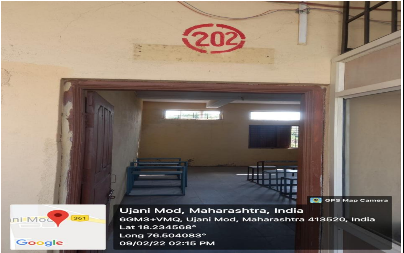
Class Room No. 202 (External view)
