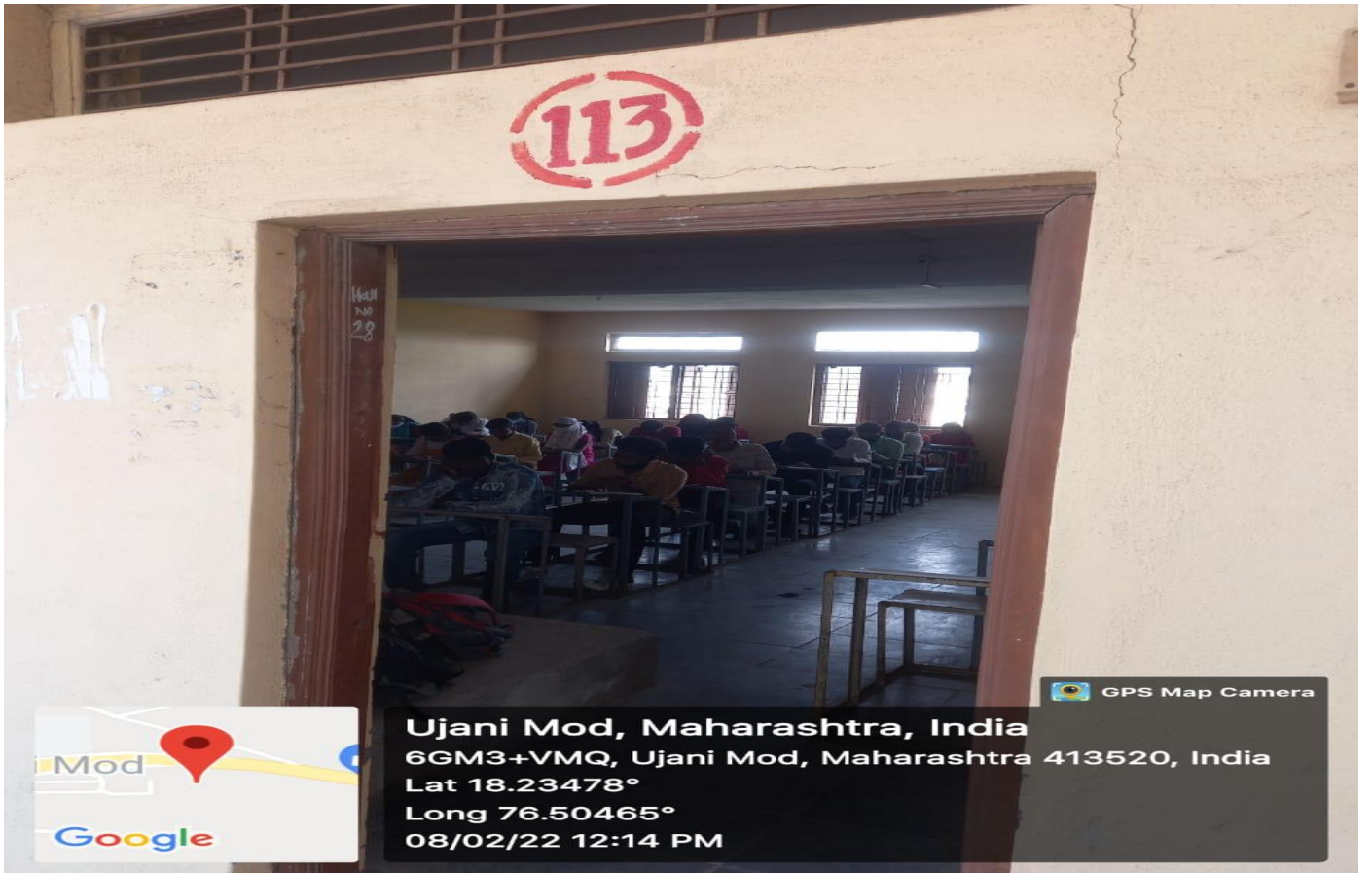
Class Room No. 113 (External view)
