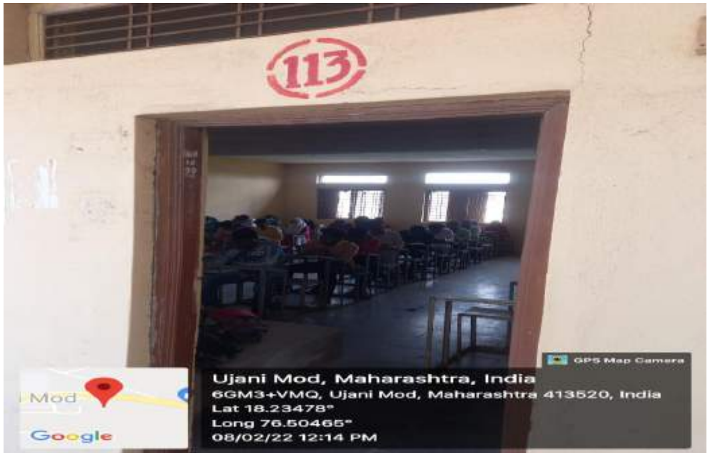
Class Room No. 113 (External view)
