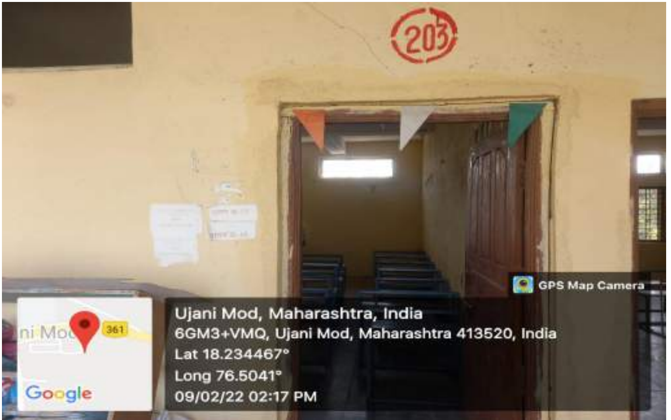
Class Room No. 203 (External view)
