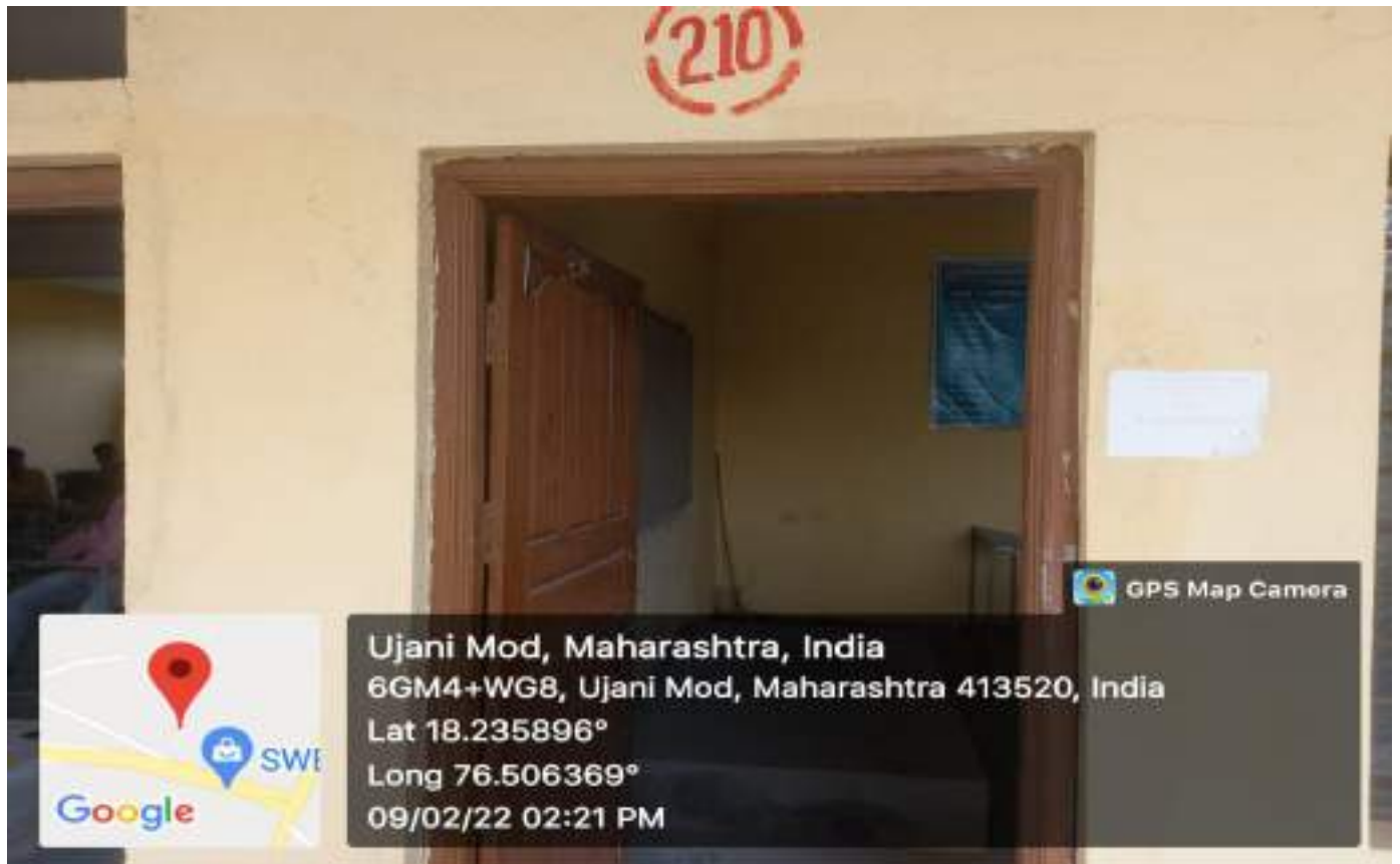
Class Room No. 210 (External view)
