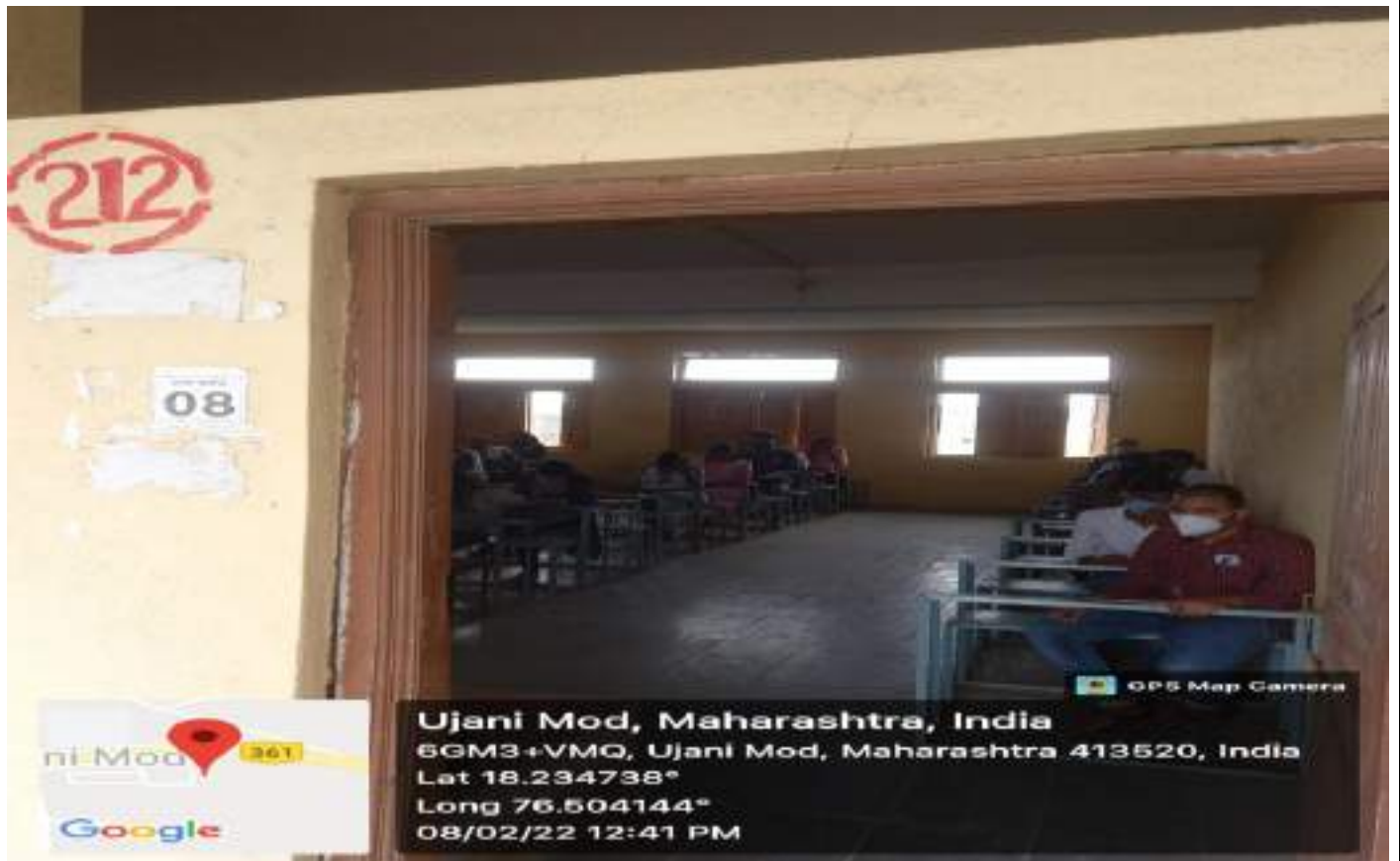
Class Room No. 212 (External view)
