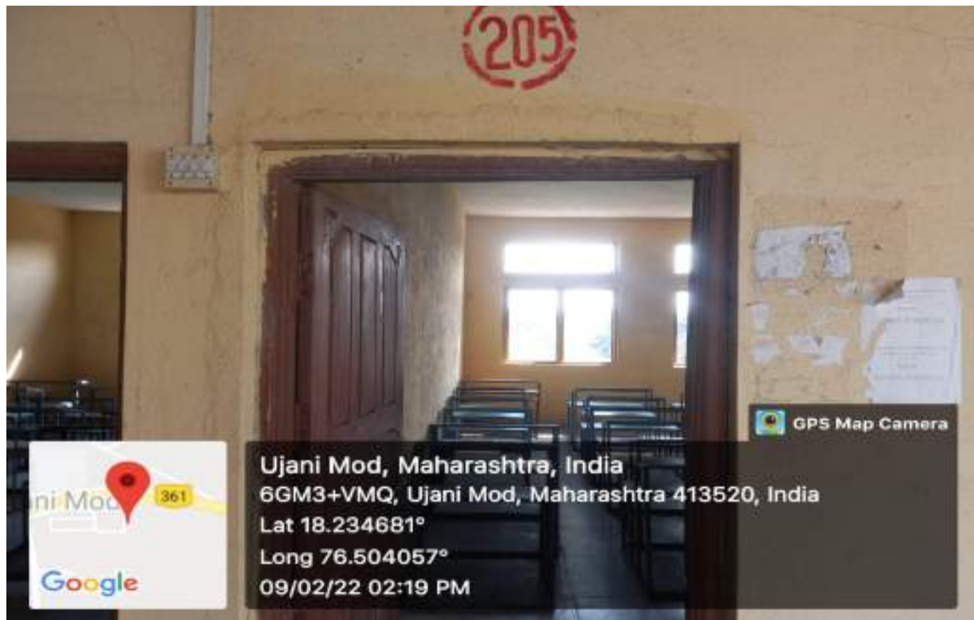
Class Room No. 205 (External view)
