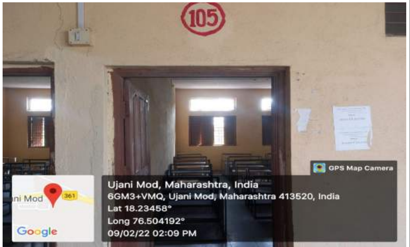
Class Room No. 105 (External view)
