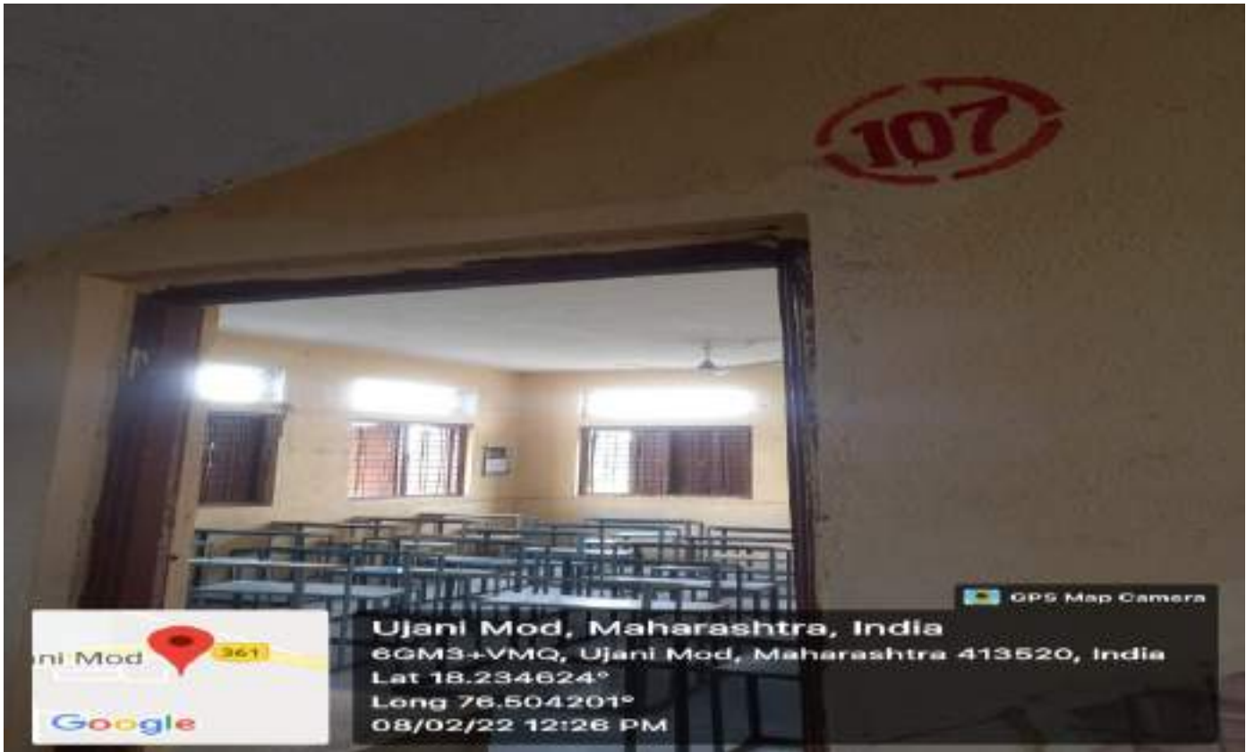
Class Room No. 107 (External view)
