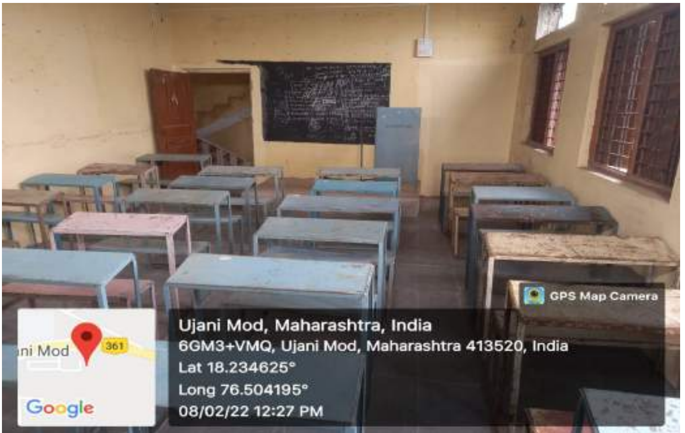
Class Room No. 107 (Internal view)
