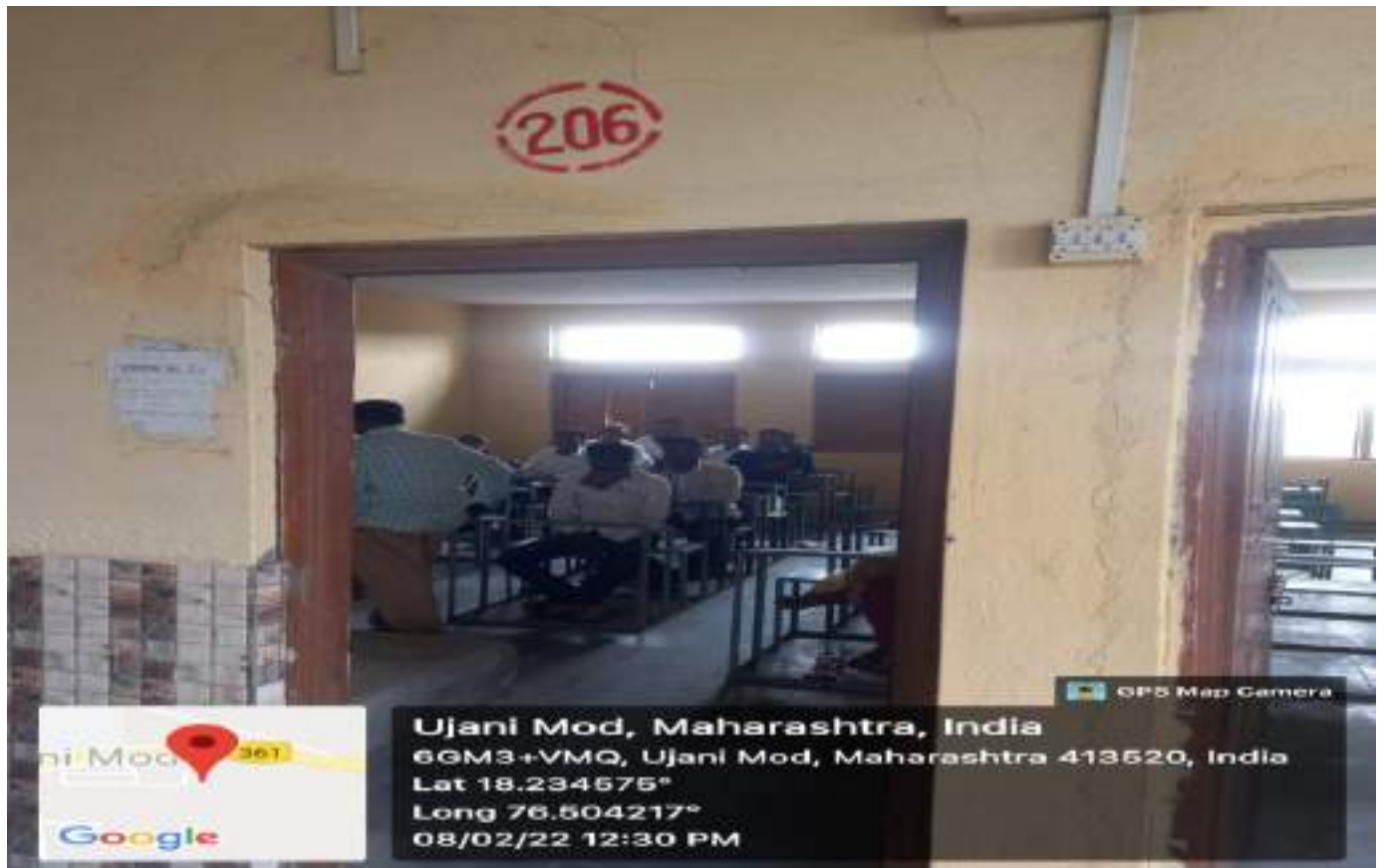
Class Room No. 206 (External view)
