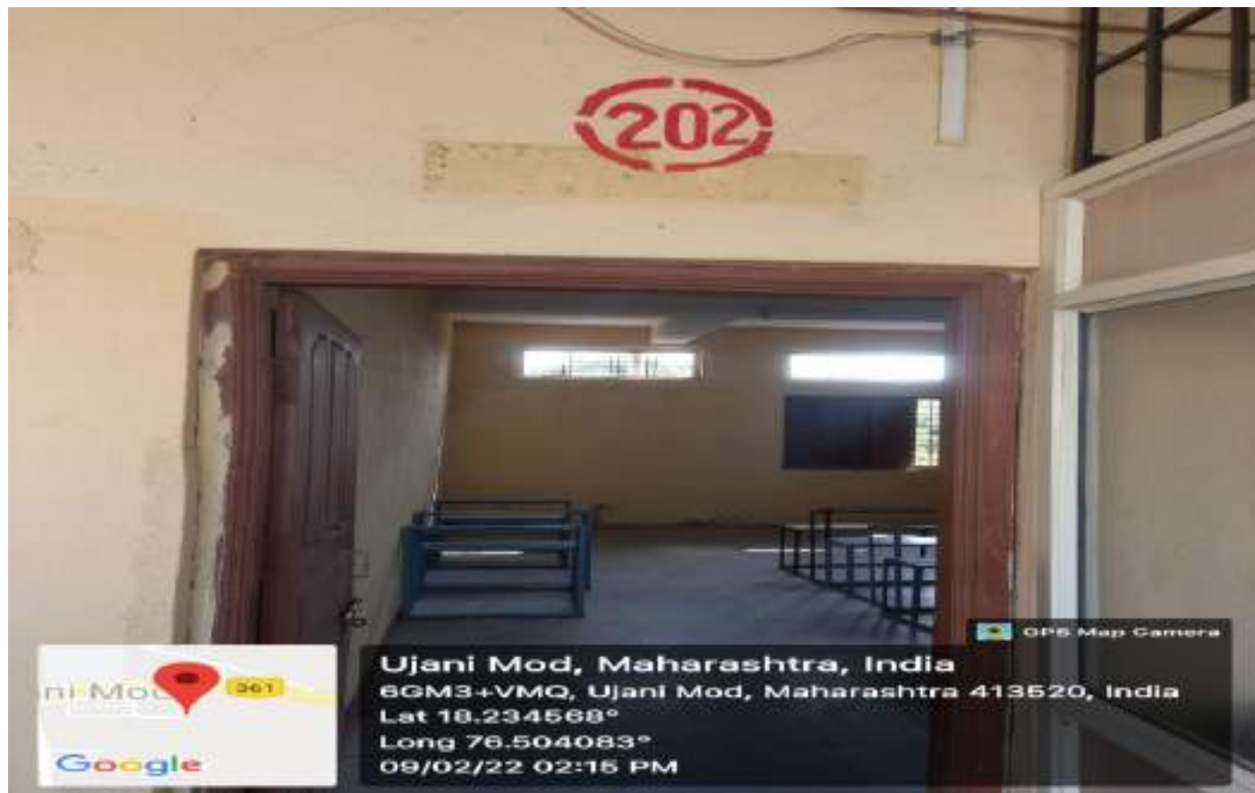
Class Room No. 202 (External view)
