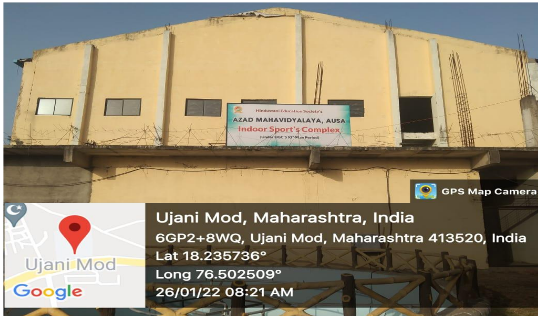
Front View of Azad indoor Sports Complex situated on North side of National Highway in campus II
