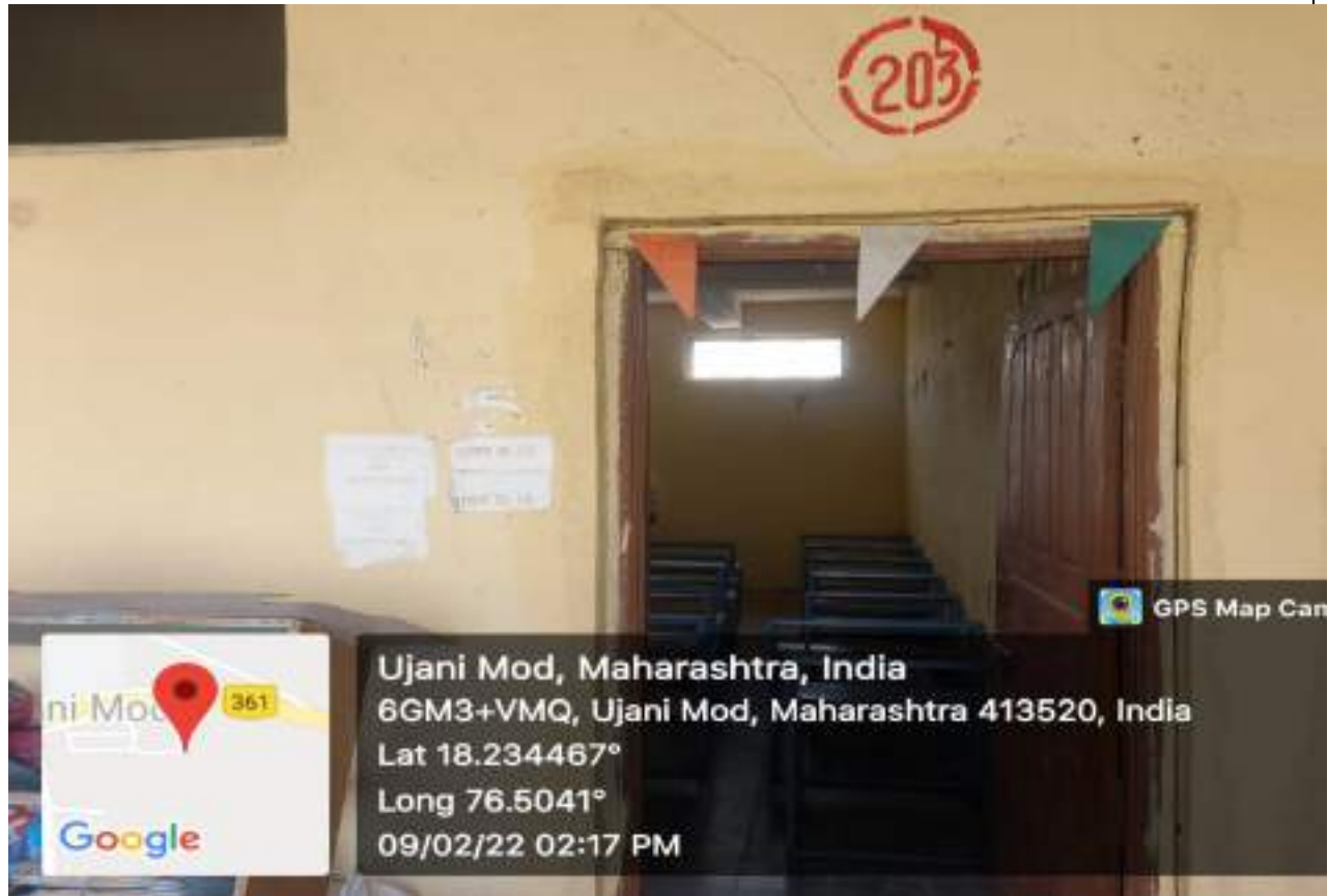
Class Room No. 203 (External view)
