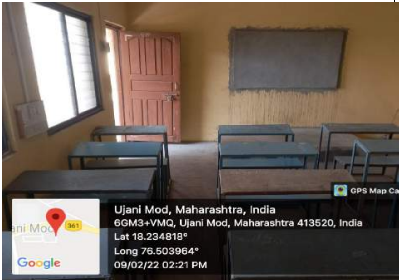
Class Room No. 210 (Internal view)
