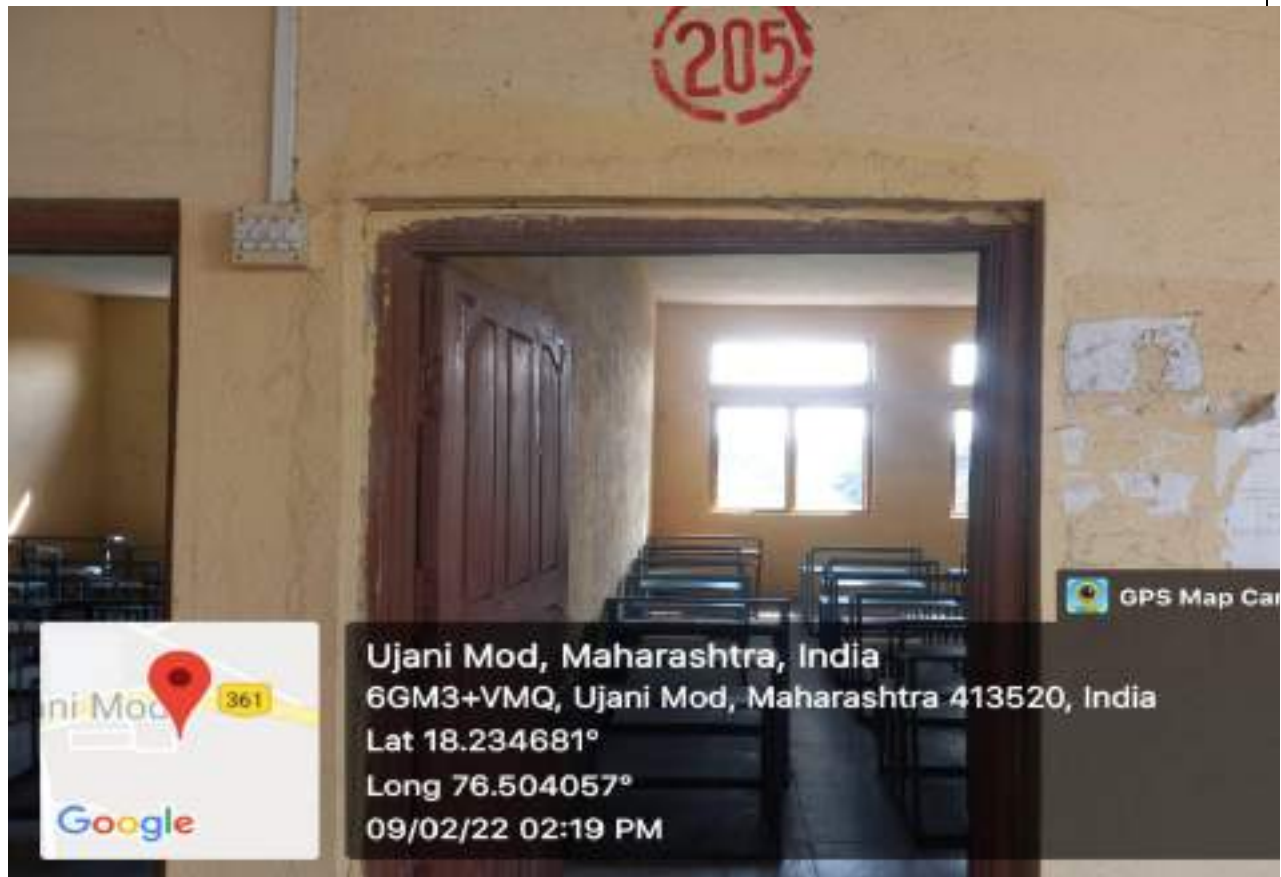
Class Room No. 205 (External view)
