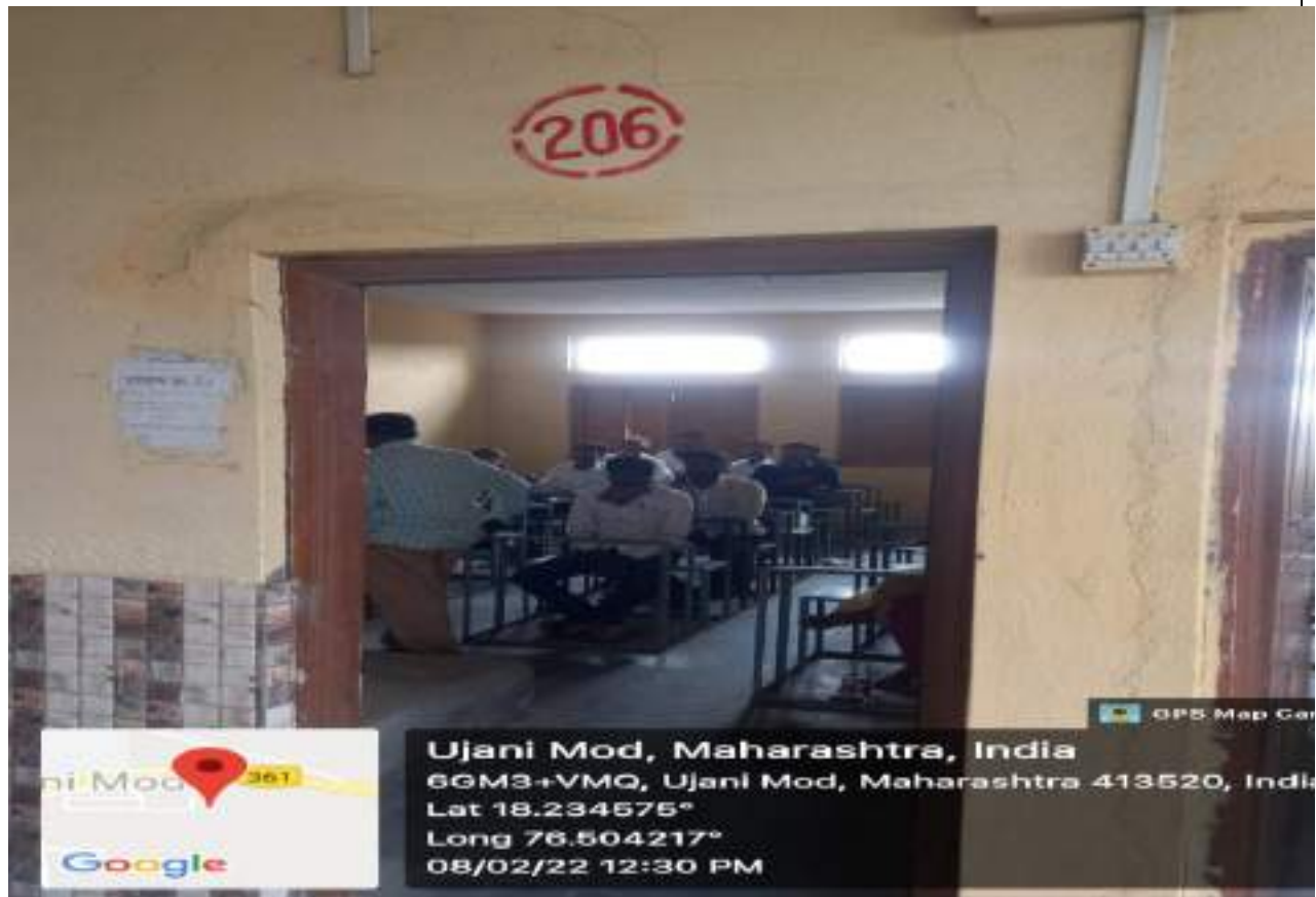
Class Room No. 206 (External view)
