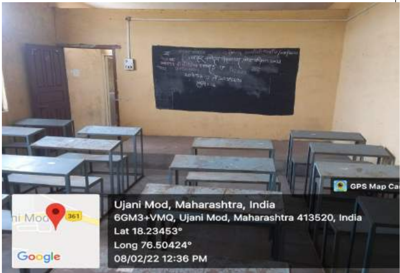
Class Room No. 209 (Internal view)
