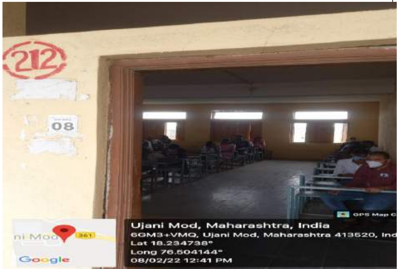
Class Room No. 212 (External view)
